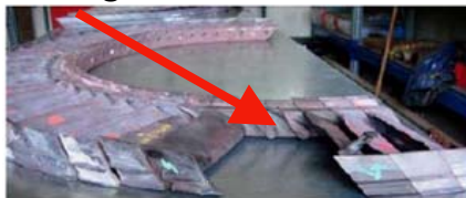
Missing blades on rotor
