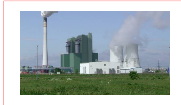
Build & operate for 3rd party: Schkopau
