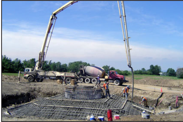
Concrete Foundation Preparation
