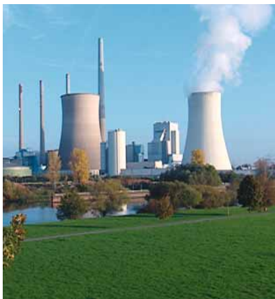
Coal-fired power station // Staudinger (GER)
