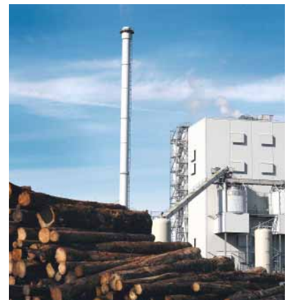
Biomass power plant // Lockerbie (GB)
