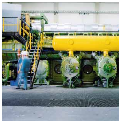
Gas storage // Our storage facilities help ensure a secure supply of gas.
