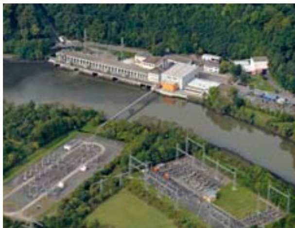
Pumped-storage power plants like this one in Waldeck, Germany, represent a good way of storing electricity for later consumption.
