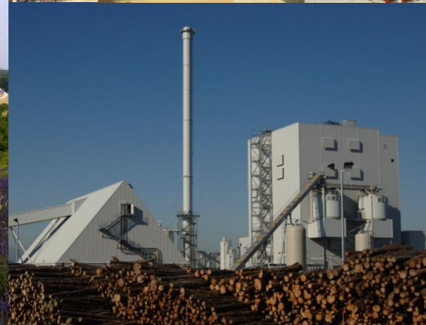
Biomass plant Steven's Croft, UK (43 MW)
