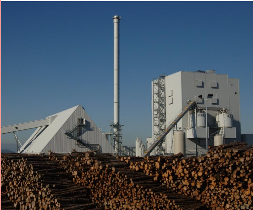
Biomass plant Steven's Croft in Scotland (43 MW, COD 2008)
