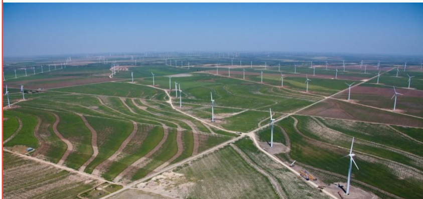
Roscoe, Texas, the world's largest onshore wind park (782 MW)
