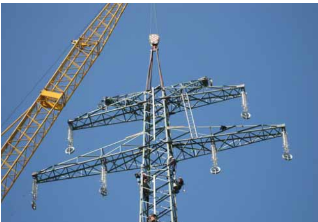
Upgrading the overhead-lines
