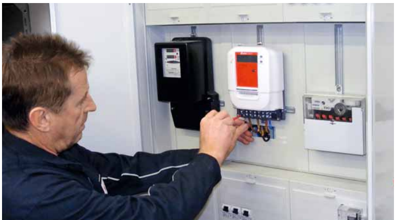
Installation of smart meter technology
